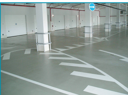
Markings road ways
